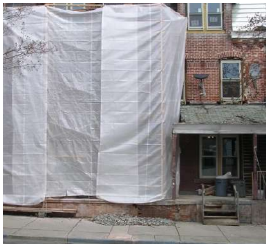
Facade Renovation to Allentown Home
