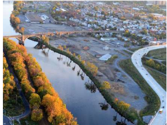
Gateway at Tilghman Street Bridge
