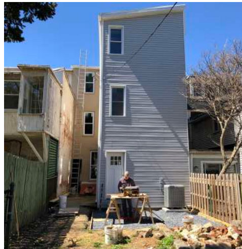
Habitat for Humanity Renovation Project Source: City of Allentown
